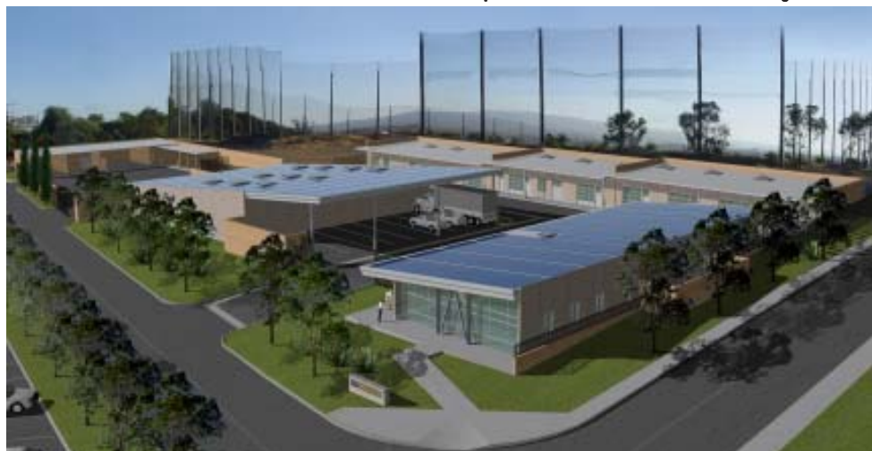
Facilities Operations and Maintenance Building
