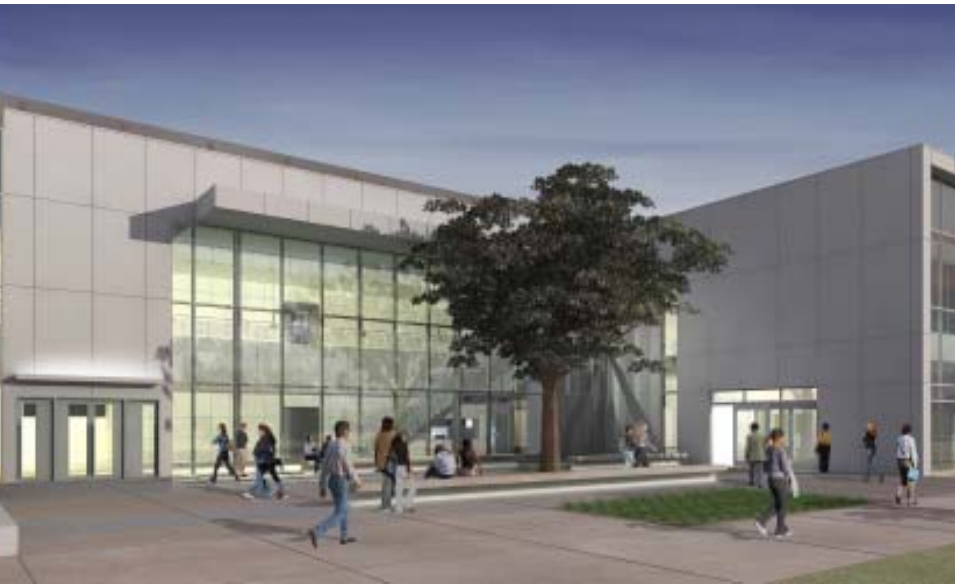
Courtyard Technology Building
