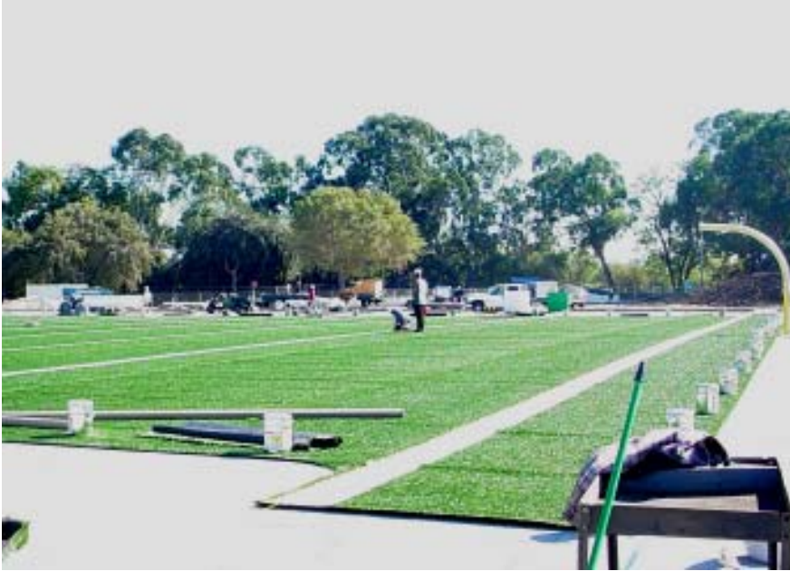
Construction on the new Track & Field
