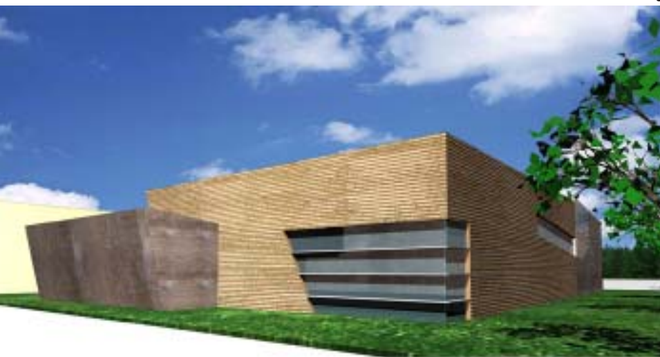
Central Plant Building
